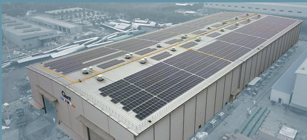
In April 2021 our tooling factory in Taicang, China installed solar panels on their rooftop. Between installation and December 2021, this system has allowed us to generate 0.97M kWh of renewable electricity, saving 390.56 tons of coal, and reducing CO<sub>2</sub> emissions by 1 050 tons.
